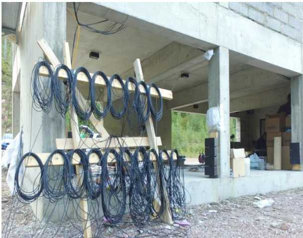
Ready to cable high frequency sensors (left) & the strain wireless module (right)
