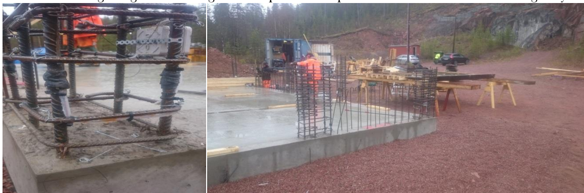
Strain sensors installation to the building's rebars
